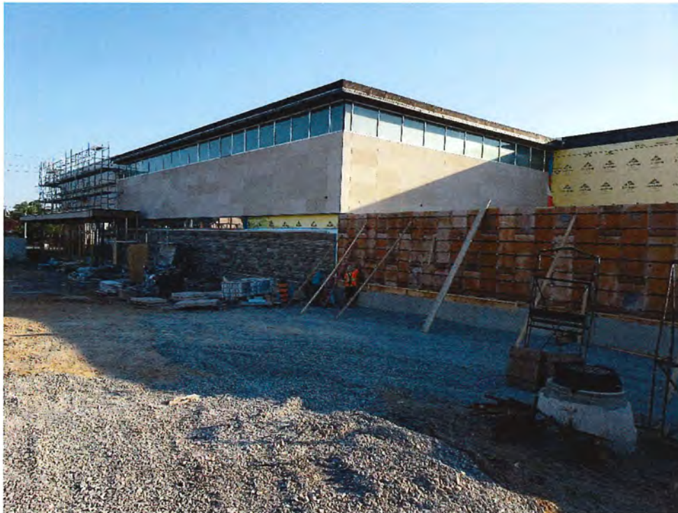
West Elevation (looking east) – Continued formwork for new security retaining wall
