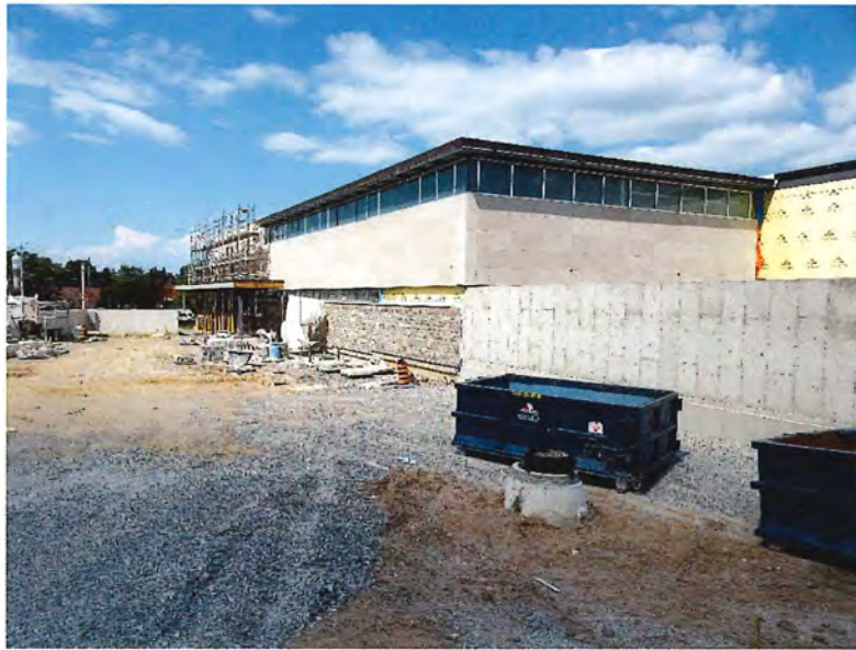
West Elevation (looking North) – complete retaining wall and removal of masonry scaffold
