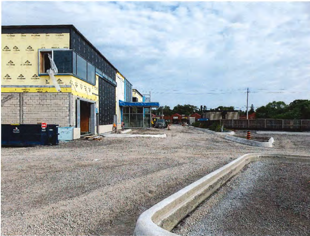
Start of Concrete Curbs – East Elevation
