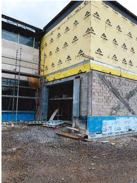
South/West Elevation (looking east) – Installation of galvanized overhead door frame
