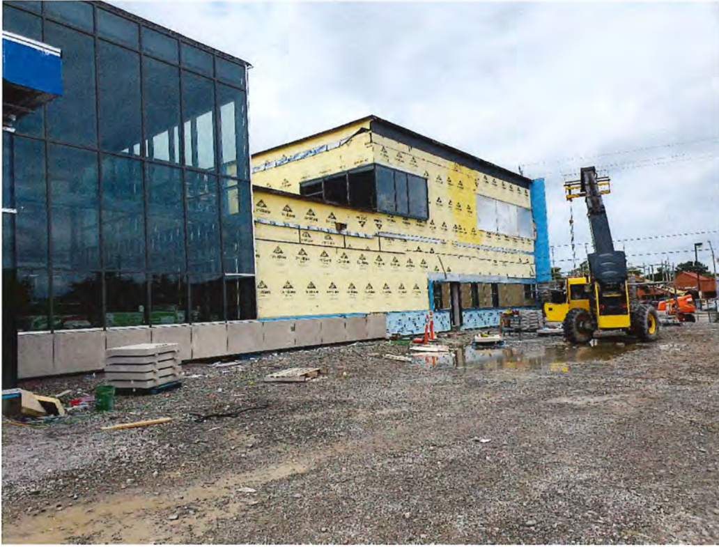
Installation of new bottom course stone panels – East Elevation
