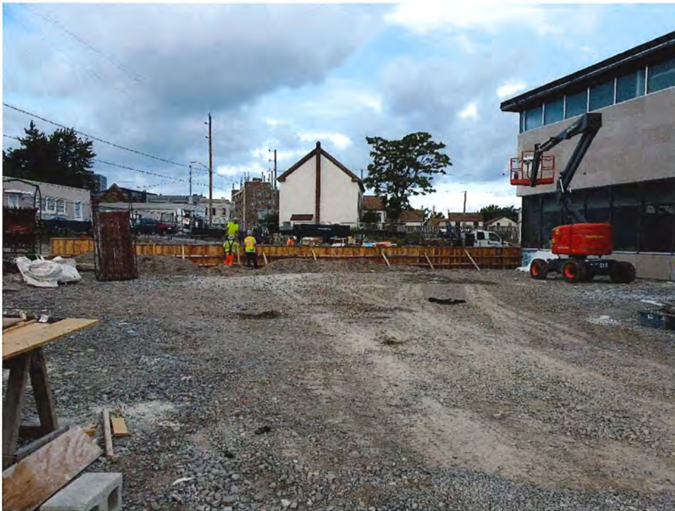
East Elevation (looking West) – Formwork for new security retaining wall
