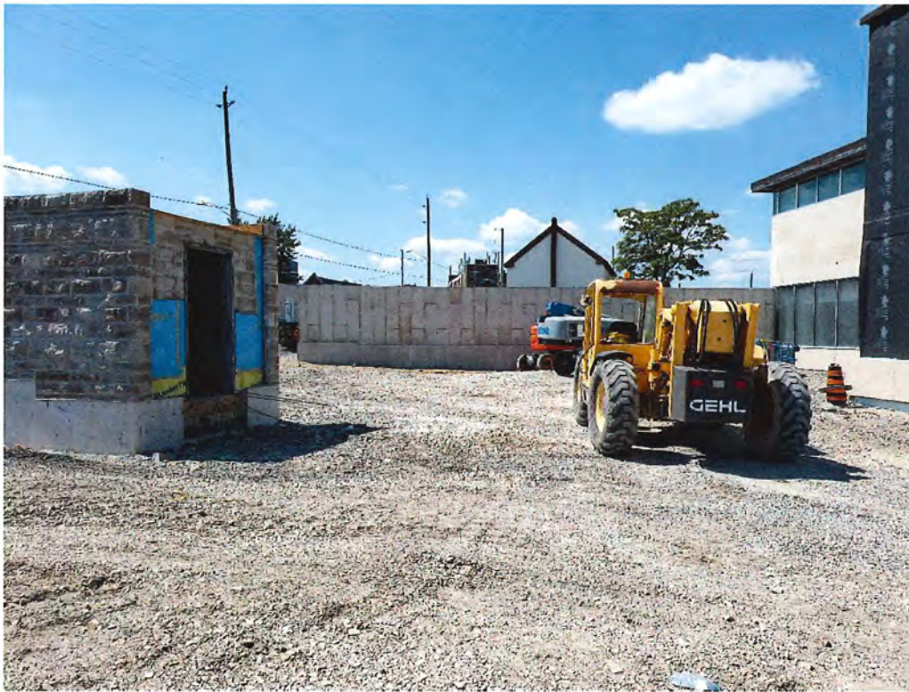
West Elevation (looking East) – poured concrete security retaining wall
