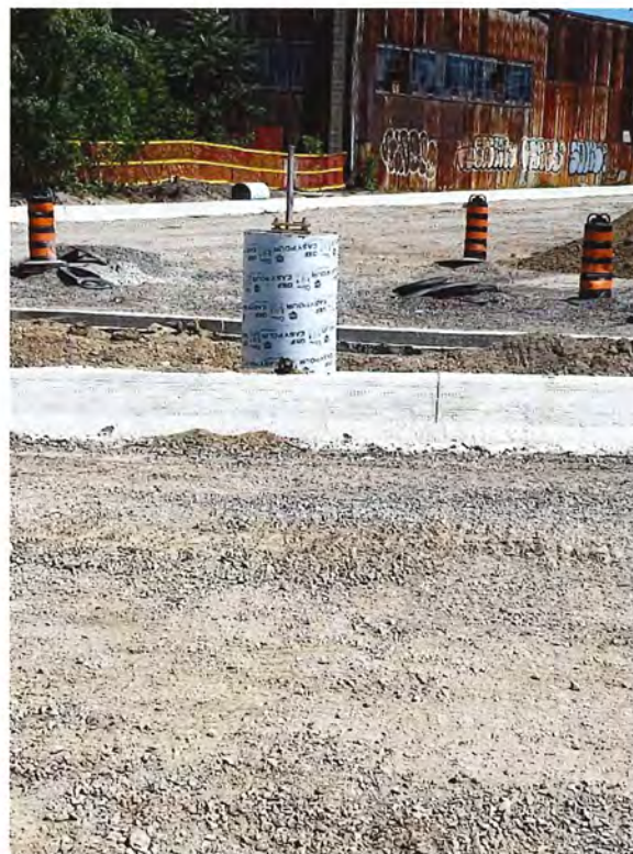
Typical sonotube light standard base
