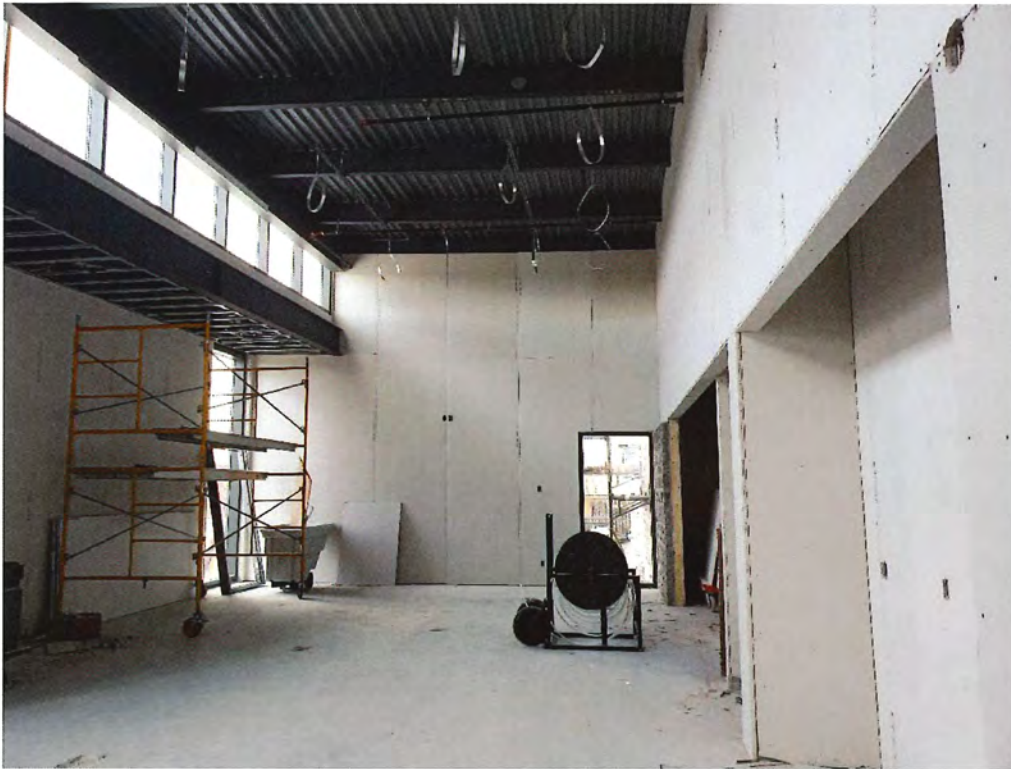
Community Mtg. Rm. – drywall complete – ready for taping & sanding
