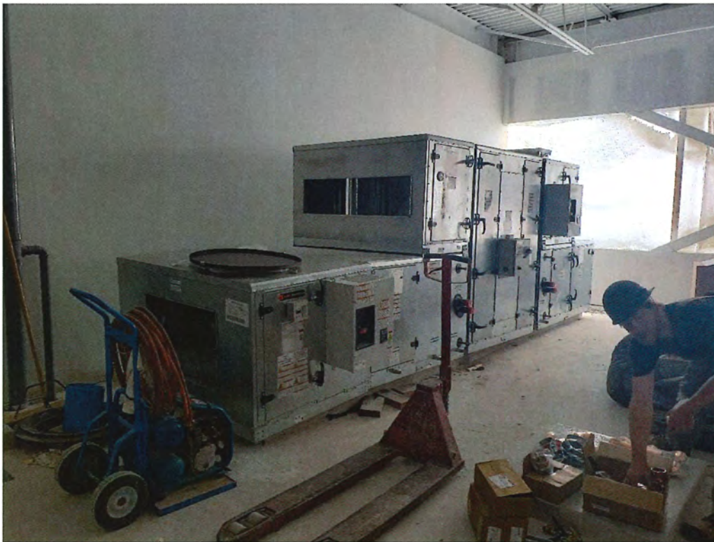
2 nd Floor Mechanical Rm. – Panel Make-Up Air Unit
