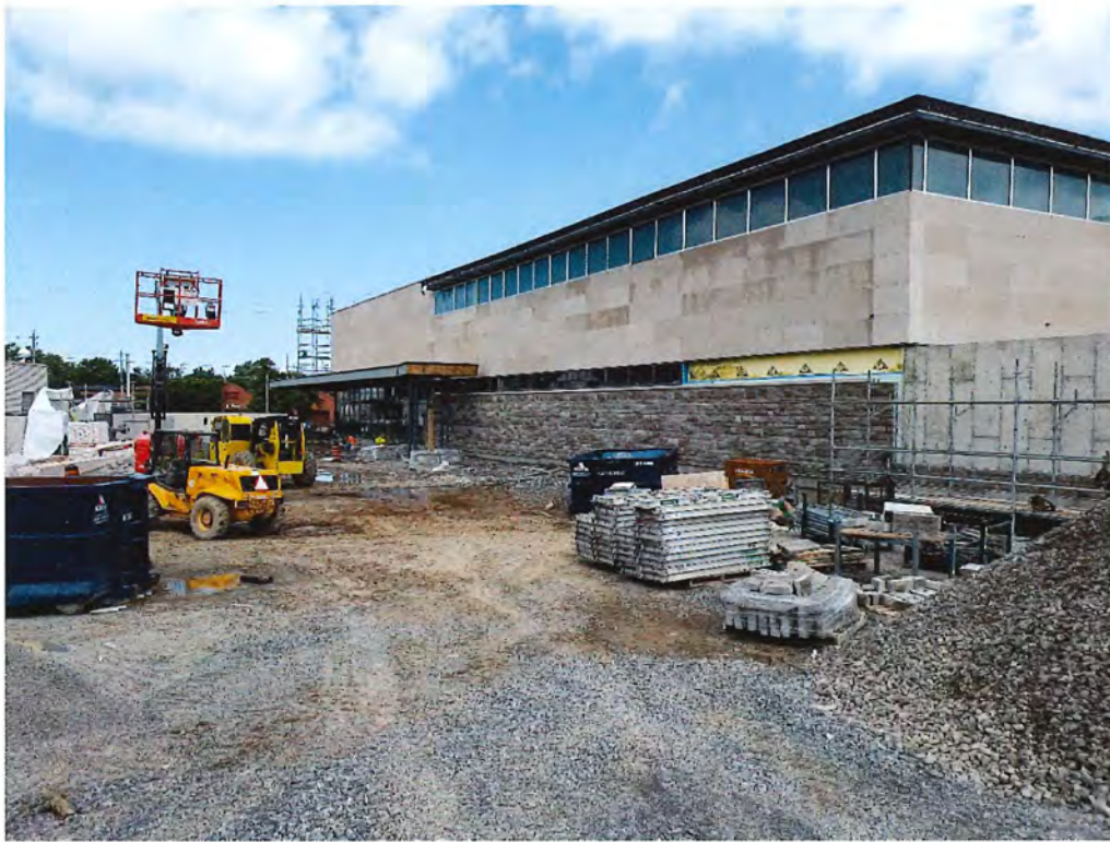
West Elevation – Commencement of Limestone install at security retaining wall
