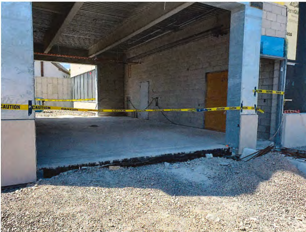
SallyPort – East Entry Door – Installation of concrete floor slab
