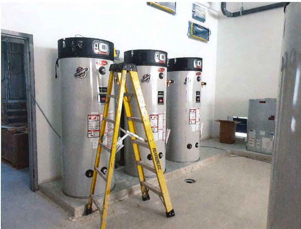
2 nd Floor Mechanical Rm. – New Gas Fired Water Heaters
