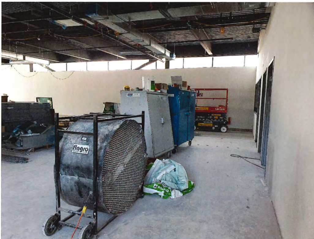
Criminal Investigations Room – Drywall taped and sanded – prepped for primer coat
