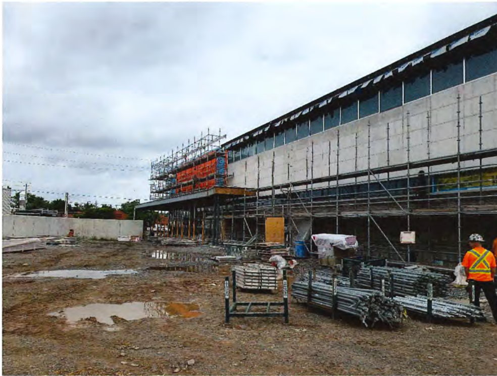
West Elevation – 80% complete upper stone panels (removal of scaffolding)
