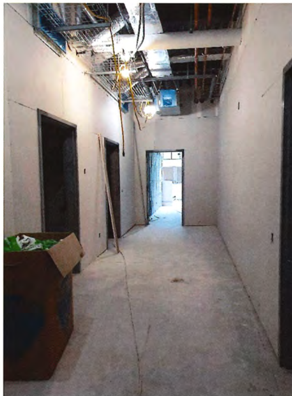
South end corridor leading to Sallyport – Drywall install – prepped for taping & sanding
