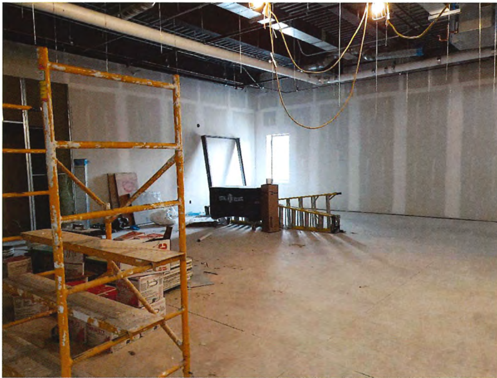
Parade Rm. – Drywall prepped and sanded – ready for primer coat
