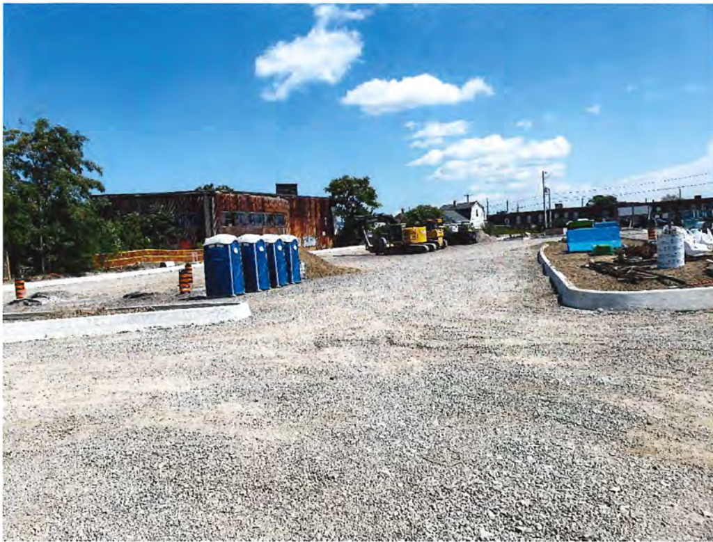
East Elevation (looking toward Niagara St.) – completed curbs and light standard bases
