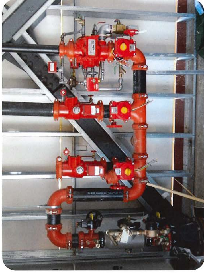
Ground Floor – Fire control system, these auto valves control water going to the fire suppression systems in the building.
