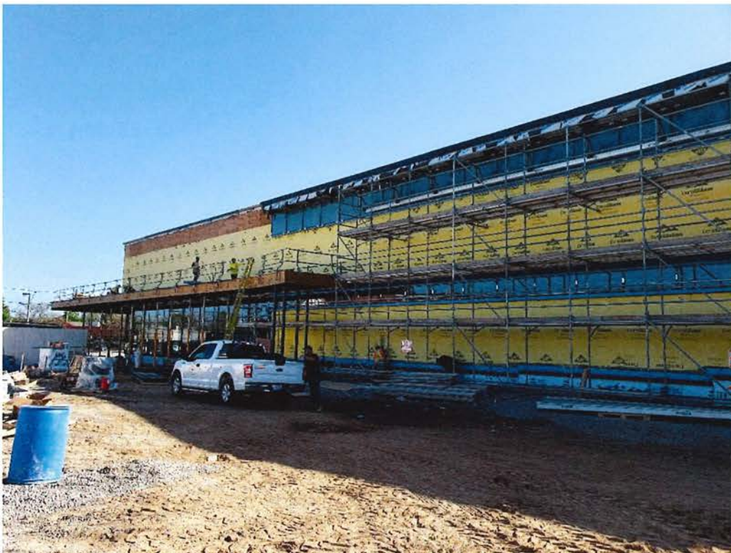
Scaffold installation along West Elevation - (commencement limestone installations)
