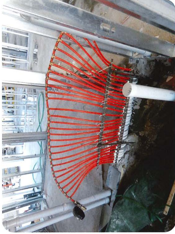
Ground Floor – showing under floor glycol heating tubes
