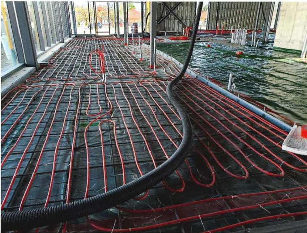
In floor radiant heat piping installations (ground floor front lobby and community room)
