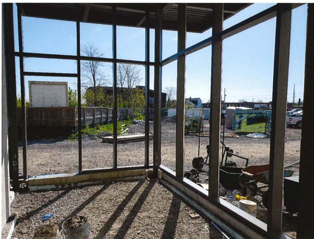
Curtain Wall Framing – East Elevation – New Staff Entry/Exit Vestibule
