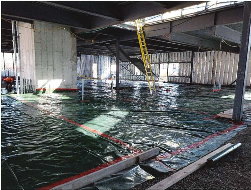
Ground floor 10 mil poly installations – (prep for future concrete slab pour)
