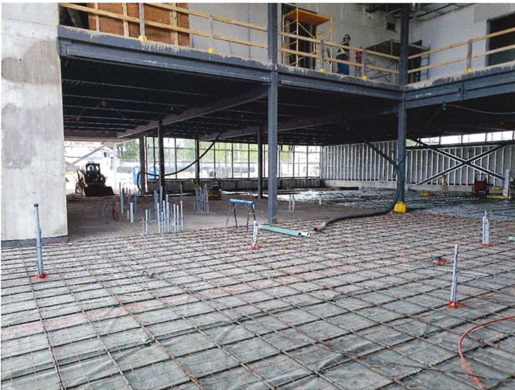
Poly & reinforcement prep for 2 nd ground floor slab pour (looking south)
