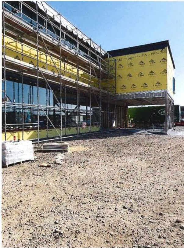
Scaffold installation along South Elevation - (commencement limestone installations)
