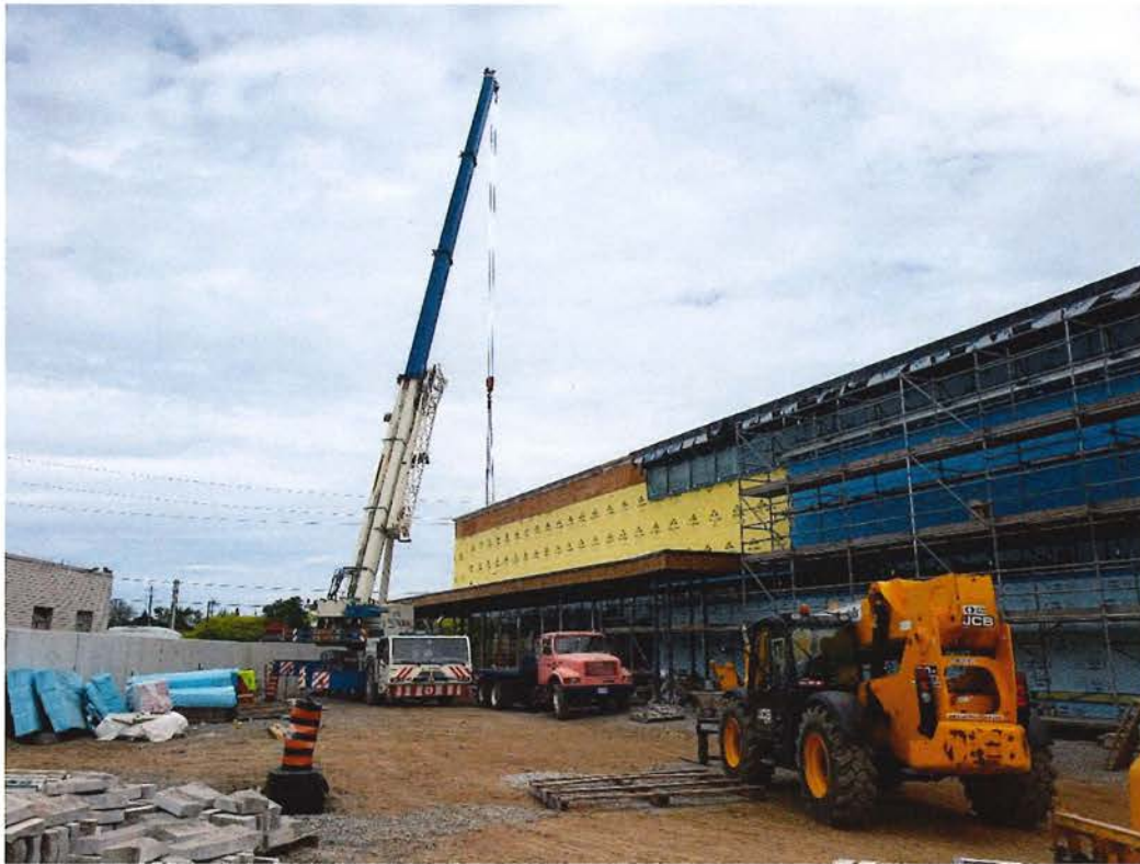
Successful crane installations of new RTU (roof top unit) & Gas Generator (looking north)
