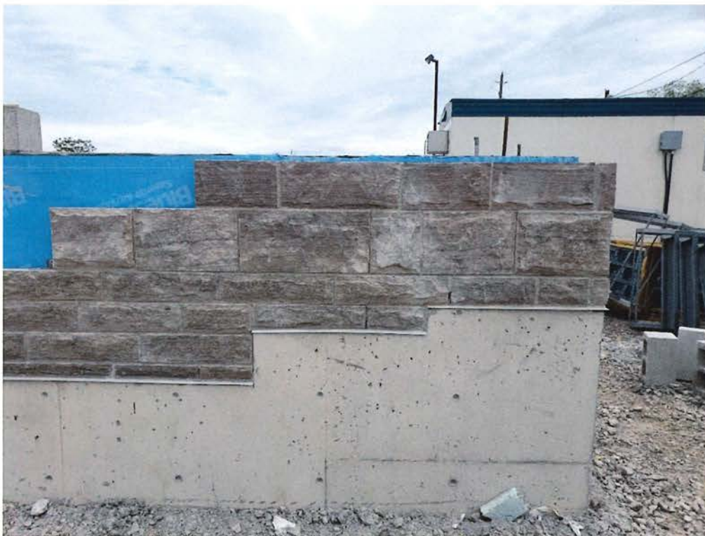
Exterior Shed – Approved Limestone installation Mock –Up
