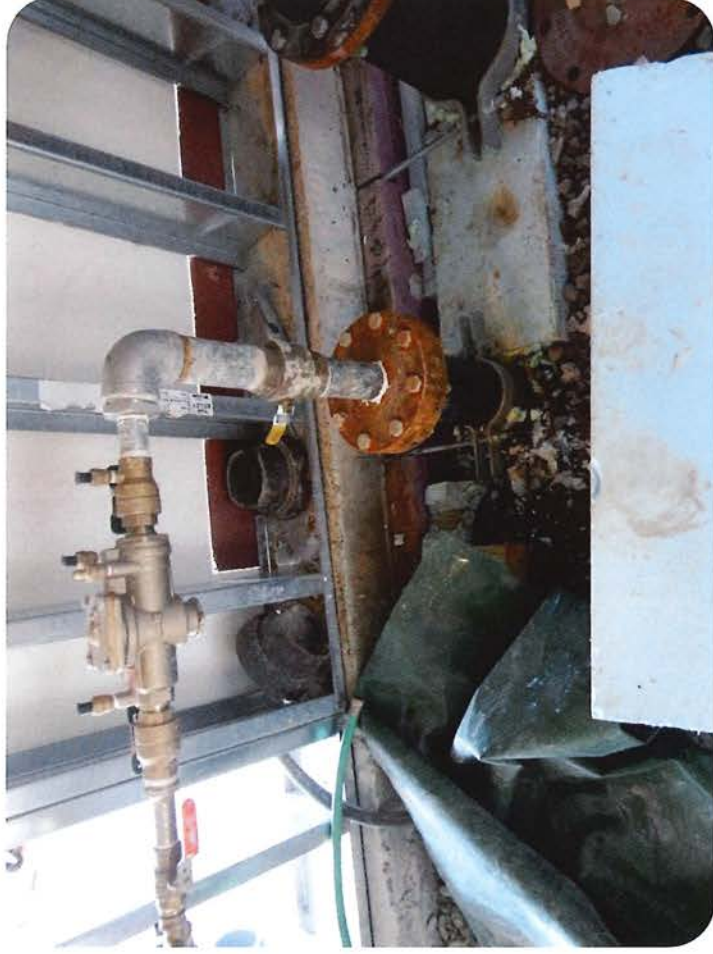
Ground Floor – showing main waterline into the building
